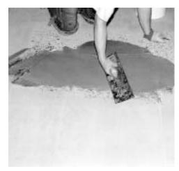
"It's thin, it gets in, and it won't pop out." Roadware 10 Minute Concrete Mender uses Microdowling<sup>TM</sup> action to repair concrete permanently.
